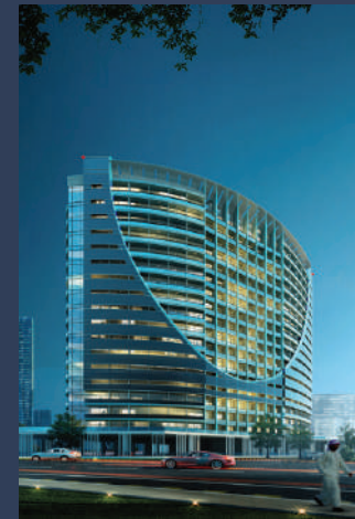
The V Tower
